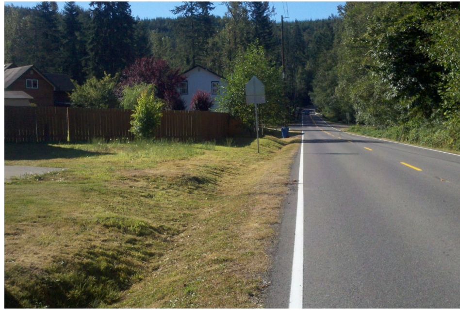
South Church Street Path: Existing
