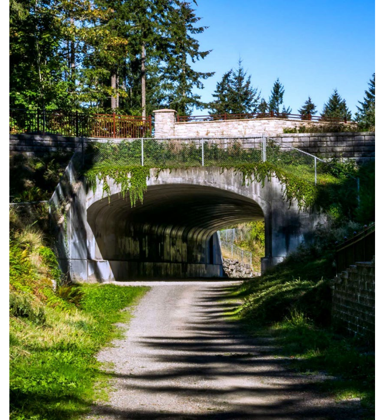
Near Lake Wilderness Park - Maple Valley, WA Green to Cedar Rivers Trail at Witte Road SE.
