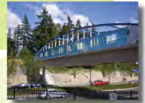
The Interurban Trail crossing Aurora Avenue.
