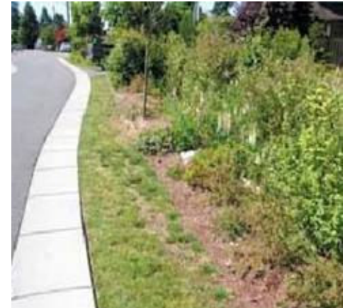
Bio-Swale next to neighborhood street
