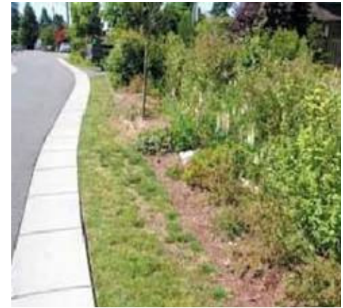
Bio-Swale next to neighborhood street
