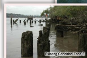
Existing Condition Zone E
