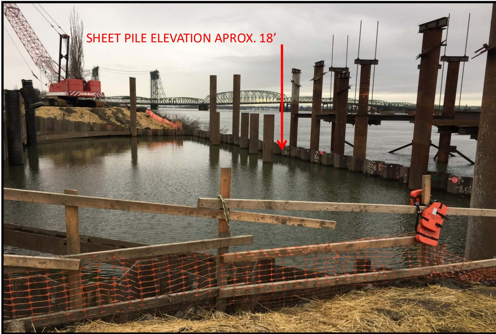
HIGH WATER AND STILL RISING. HAD TO START OVER WITH THE PUMPING. MARCH 13, 2017
