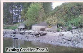
Existing Condition Zone A
