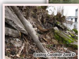
Existing Condition Zone D
