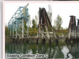
Existing Condition Zone C
