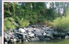
Existing Condition Zone D
