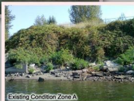
Existing Condition Zone A
