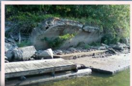
Existing Condition Zone C
