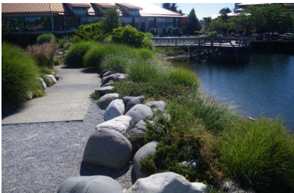
Flood protection and shoreline enhancement through habitat design Source: City of Olympia Engineered Response to Sea Level Rise
