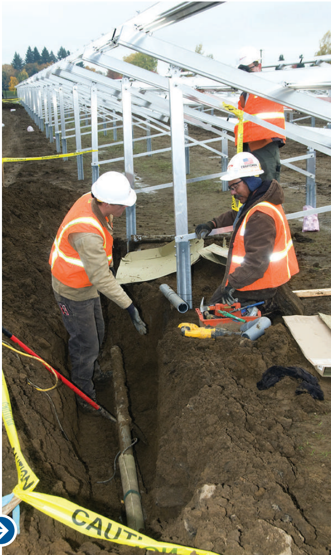
Workers ensuring frames for solar panels have a good foundation. (By Oregon Department of Transportation. "Footings" uploaded by Smallman12q. Licensed under creativecommons.org/licenses/by/2.0 )
