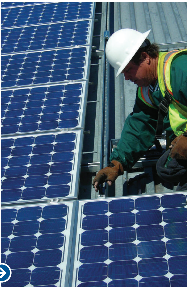
A construction worker installs solar panels at the Marine Corps Air Ground Combat Center in Twentynine Palms, California.
